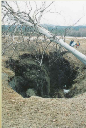
Thermokarst pit in farm field near Fairbanks gives perspective to damage that melting ice lenses can do.
