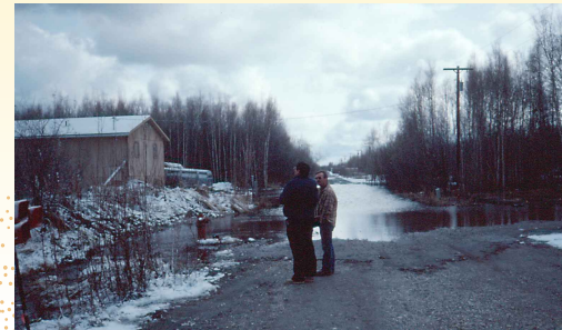
Localized flooding can happen when fill and debris clog surface drainage ways.
