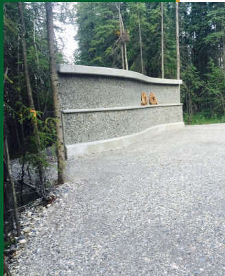
Progress is being made on North Pole Memorial Park
