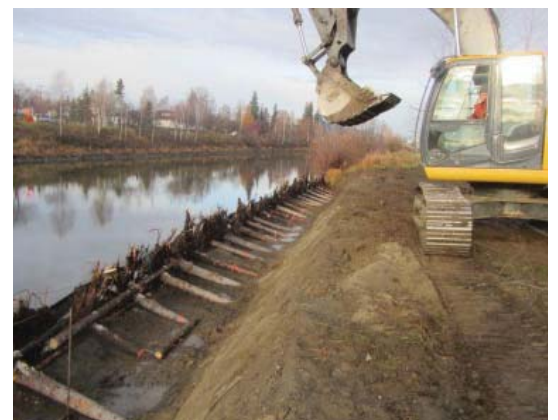
FNSB building root wad project during construction
