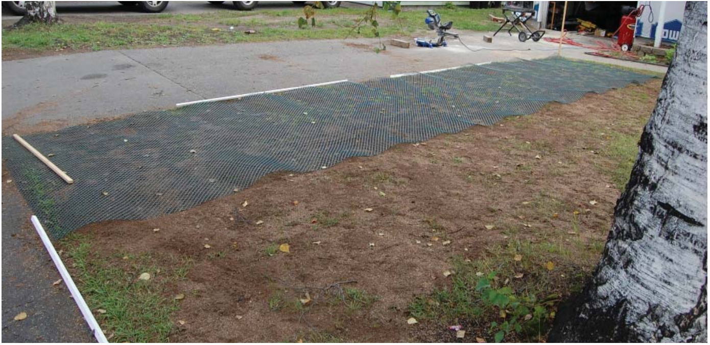
Ground leveled, with mesh laid out prior to pinning.
