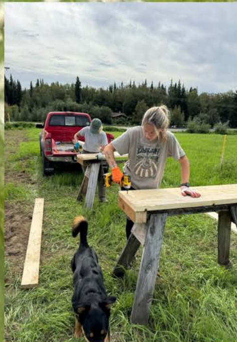
Liz Kempton and Ann Rippey building garden boxes for the Native Plant Project.
